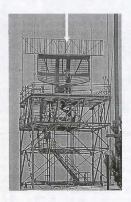
There are two types of radar antennas. Type 1 has a rotating external visible antenna. If the antenna is rotating, the system is active. "Only become exposed as long it takes to walk by, and walk as far away as possible".
