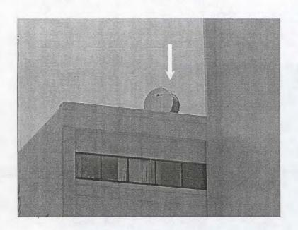
This is an example of a microwave antenna on a building rooftop. Microwave antennas, or dishes are directional and pose little danger from behind or beneath, but do not stand directly in its transmission path.
