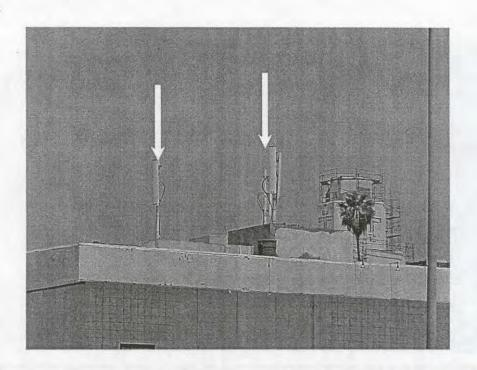
This is a smaller cellular site on Western at the Hollywood Freeway. It only has three antennas. The risk is higher than the other site because these antennas are not as elevated and direct exposure to members on the roof is greater. De-energizing the building's power will not deactivate this site as most cellular cites have generator backups. "Only become exposed as long it takes to walk by, and walk as far away as possible".
