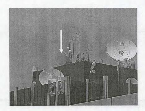
This Microwave dish poses little danger because it hangs over the penthouse wall, well over the height of a firefighter and no direct walkway in front of it. "Only become exposed as long it takes to walk by, and walk as far away as possible".
