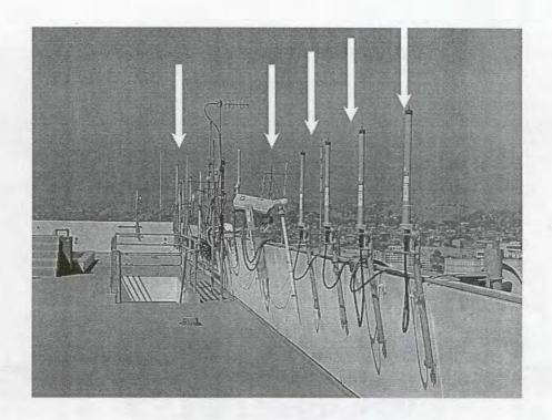
Radio antennas can also pose a health hazard with long term exposure. This antenna array on the roof of City Hall East demonstrates a high RF environment. This is another case of "Only become exposed as long it takes to walk by, and walk as far away as possible".
