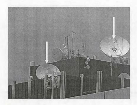
This rooftop in Hollywood has a good cross-section of antennas. The satellite dishes are fairly safe as they are elevated and send their signal at a high angle. "Only become exposed as long it takes to walk by, and walk as far away as possible".
