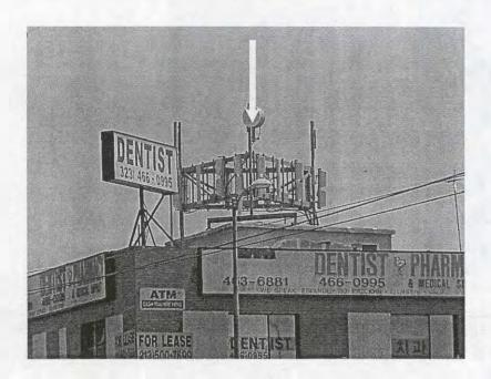
This cellular site is located at Santa Monica & Western. Members laddering, or conducting roof operations on this building should use care not to walk in front of the antenna paths. This site has the antennas slightly elevated on a penthouse. De-energizing the building's power will not deactivate this site as most cellular cites have generator back-ups. "Only become exposed as long it takes to walk by, and walk as far away as possible".
