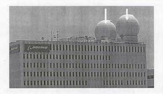
Type 2 has the rotating portion of the antenna in a dome making activity determination difficult. These domes can emit very large amounts of RF radiation and can be potentially life-threatening to approach them if they are active. Confirmation of de-energization must be made prior to roof operations commencing. This rooftop near LAX could be extremely hazardous if the radar is operational and at full power. "Only become exposed as long it takes to walk by, and walk as far away as possible".
