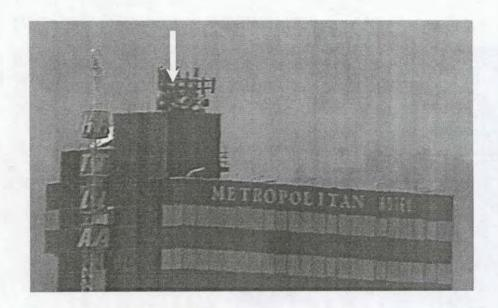
This is an example of microwave dishes & cellular antennas mounted on a hotel in Hollywood that is on a penthouse, making exposure less likely to firefighters on the roof. "Only become exposed as long it takes to walk by, and walk as far away as possible".
