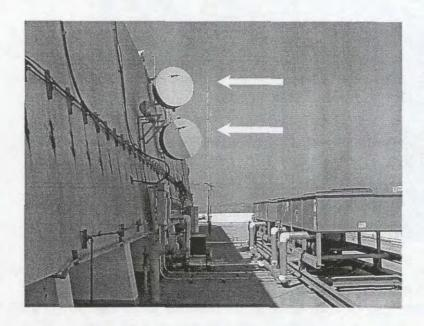
This is a photo of a microwave dishes on the roof of City Hall East. The best path to approach these dishes is close to their supporting wall, and stay underneath their transmission path. These dishes are tall enough that you can walk underneath them. "Only become exposed as long it takes to walk by, and walk as far away as possible".
