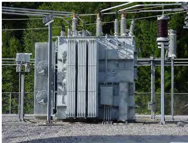
Figure 9.20: Substation transformer.
